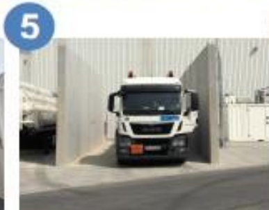
Grid injection plant
