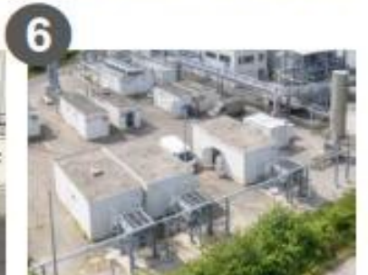
Hydrogen filling station
